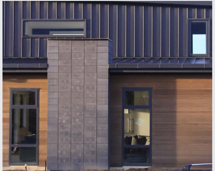
Stack bond masonry block
