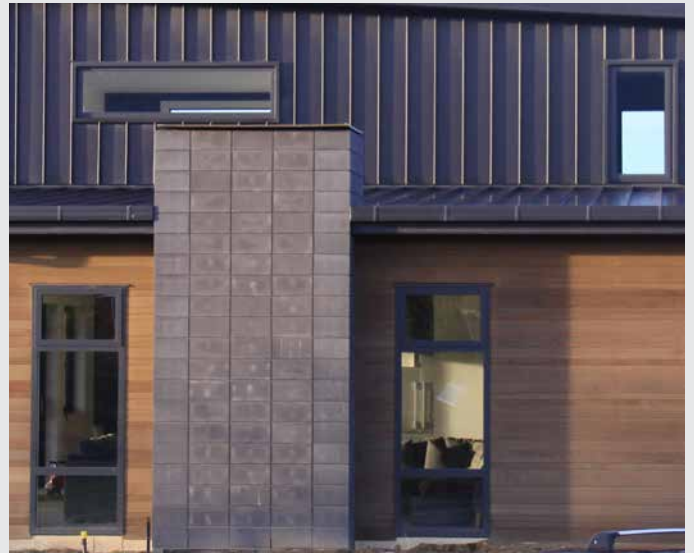
Stack bond masonry block
